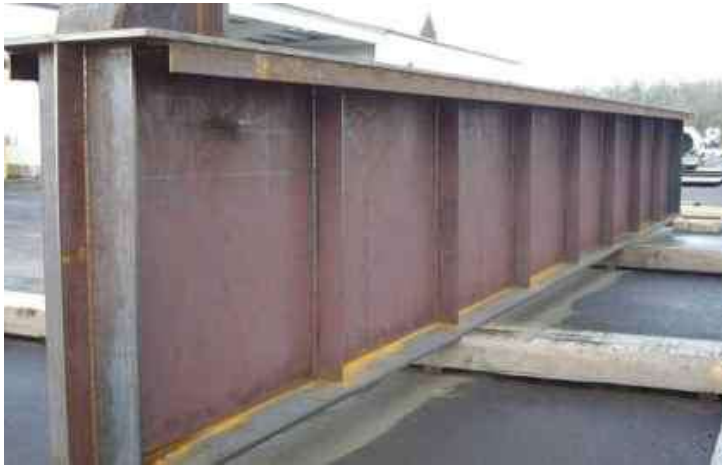
Fig 3: Plate Girder with Vertical Stiffeners
